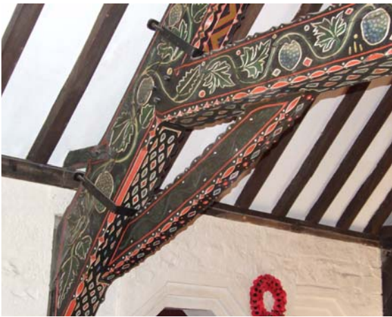
Close up of the Rood Beam decoration
