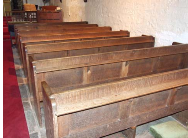
Rear view of the pews showing different style of panelling on the pew backs
