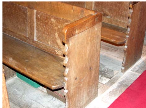
Side view of pews showing exposed tenon joints and wavy decoration on the ends of the pews
