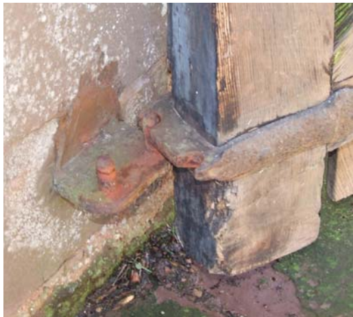
One of the Lych Gate lower gate hinges showing the novel 'double pintle' fixing (left) and the equally novel catch arrangement for the gate (right).
