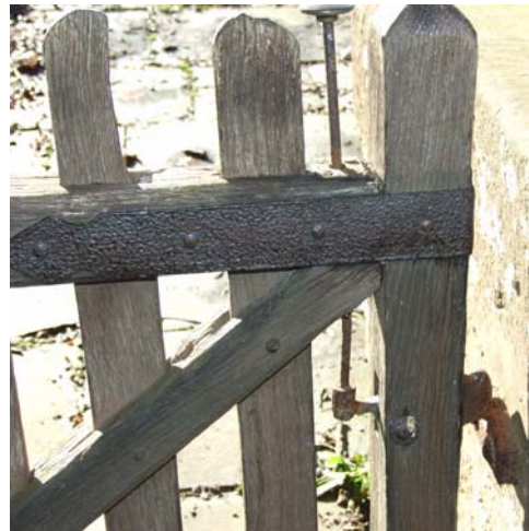
One of the Lych Gate lower gate hinges showing the novel 'double pintle' fixing (left) and the equally novel catch arrangement for the gate (right).
